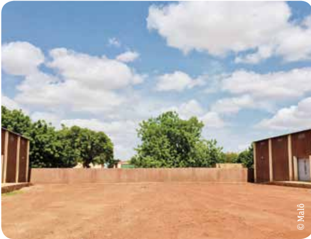
Faso Jigi's storage warehouses. Malô's rice fortification line is installed in the building on the left and unfortified rice is stored in the building on the right. (Ségou, Mali)
